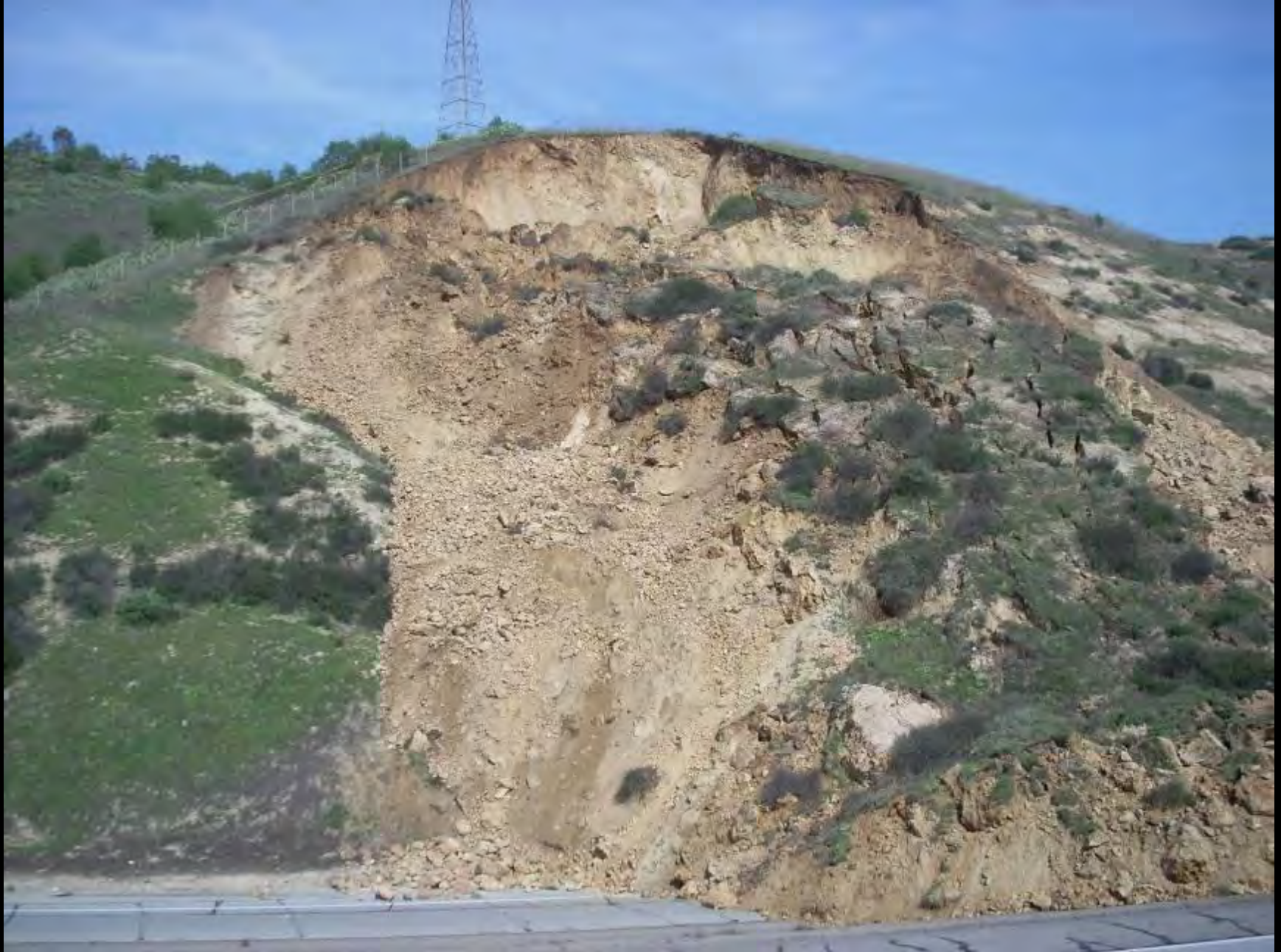
Landslide closes 57 Freeway connector, February 18, 2010
