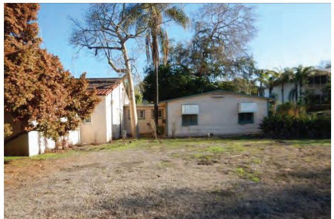
Building A-1 Mail Room
