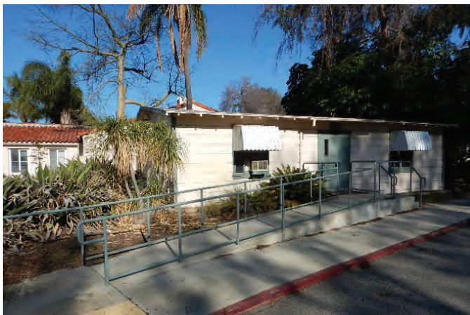
Building A-1 Mail room
