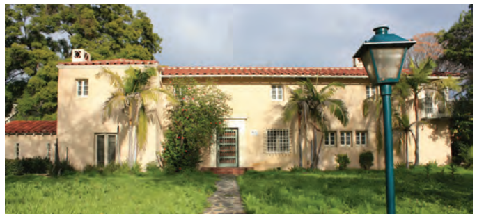
Building 60 - Research Center 1
