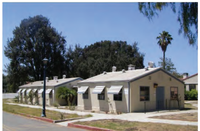
Building A-2 Southwest Elevation
