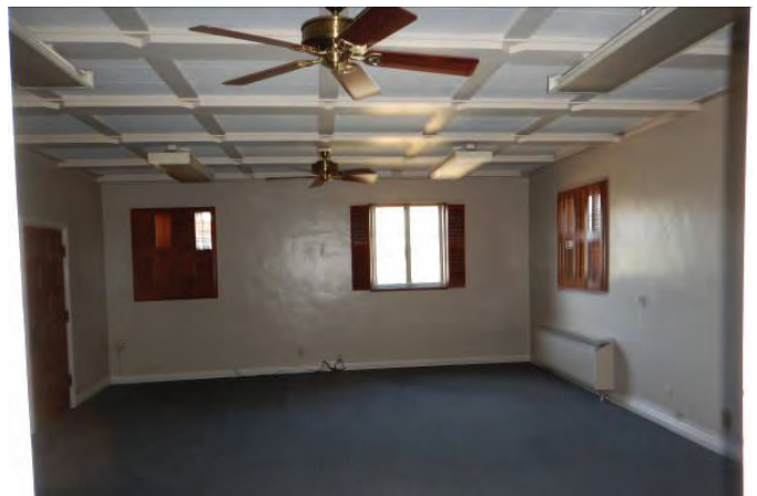
Building A-1 Interior Office
