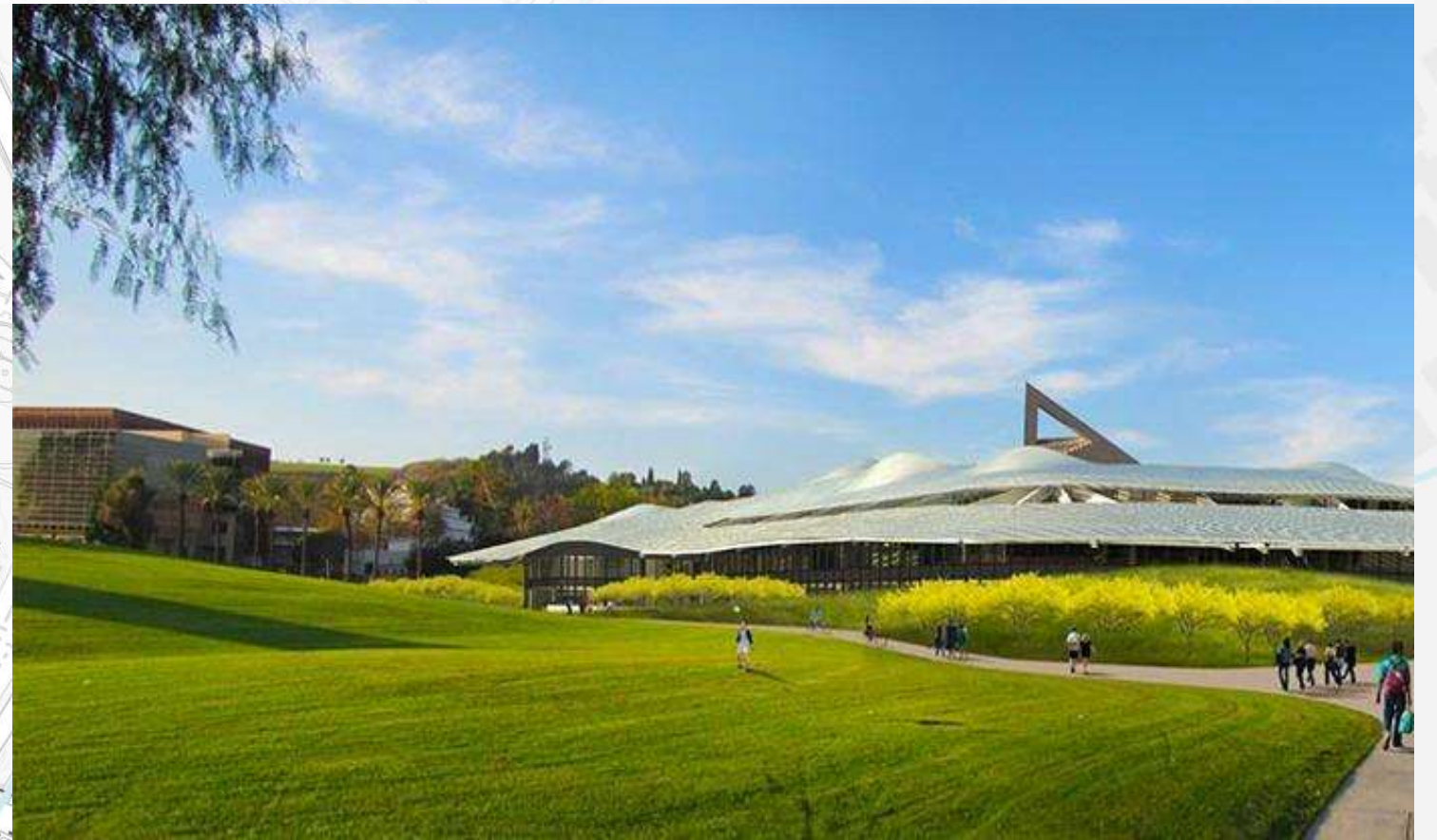
Student Services Center - under construction, open Fall 2018
