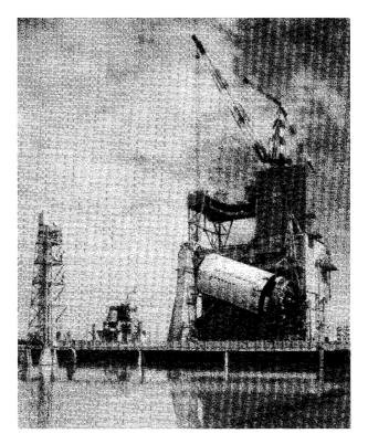
A crane hoists a section of the Saturn V rocket into place on its test stand at the Mississippi Test Facility (from the Stennis Space Center, SSC-67-701C, reprinted in Herring, Way Station to Space, p. 138).
