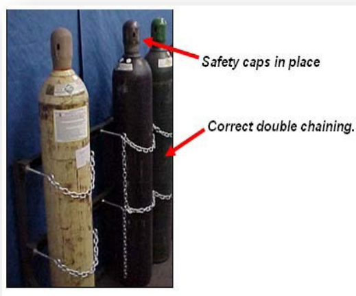
Cylinders stored and chained correctly
